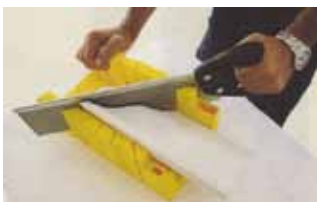
Start from one corner, cut the miters.
