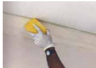
Press the moulding against the ceiling corner. Using a damp sponge clean the joint to smooth.
