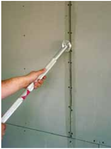
Easily and economically eliminates the drywall butt joint problem by creating a tapered edge on the butt joint.
