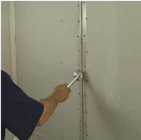
Easily and economically eliminates the drywall butt joint problem by creating a tapered edge on the butt joint.
