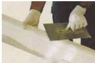
Using a commercially available gypsum base adhesive, apply a generous layer to the two flat back edges of moulding.
