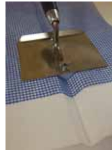
After coating your groove with base coat, place a workable width of mesh on top of the precut groove. Then move the matching groove sled forward to imbed the mesh and remove any excess base coat. The sled will push the mesh into your base coat evenly, filling the precut groove and eliminating any snags or cuts in the mesh that might occur with an ordinary trowel.
