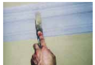
When joining the mouldings, apply a generous layer of adhesive between the pieces. Clean excess off using a putty knife. Once cured, sand joint smooth.
