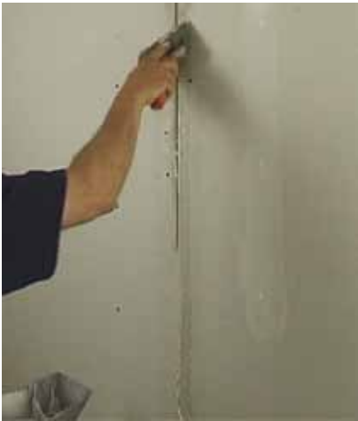
Easily and economically eliminates the drywall butt joint problem by creating a tapered edge on the butt joint.
