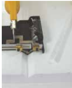
Select the appropriate cutting blade for your Hot Knife Groover. Working from predetermined markings on your substrate cut your groove in the EPS insulation.
