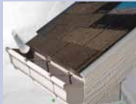
Install Exterior Wall Cladding.
